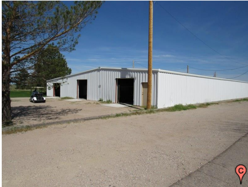
Golf Car Storage Building
